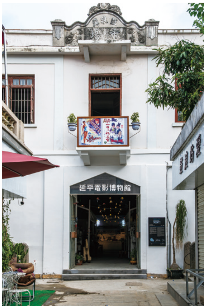
◎ 延平戏院旧址。（康伦恩 摄） Former Yanping Theatre. (Photo by Kang Lun'en)
