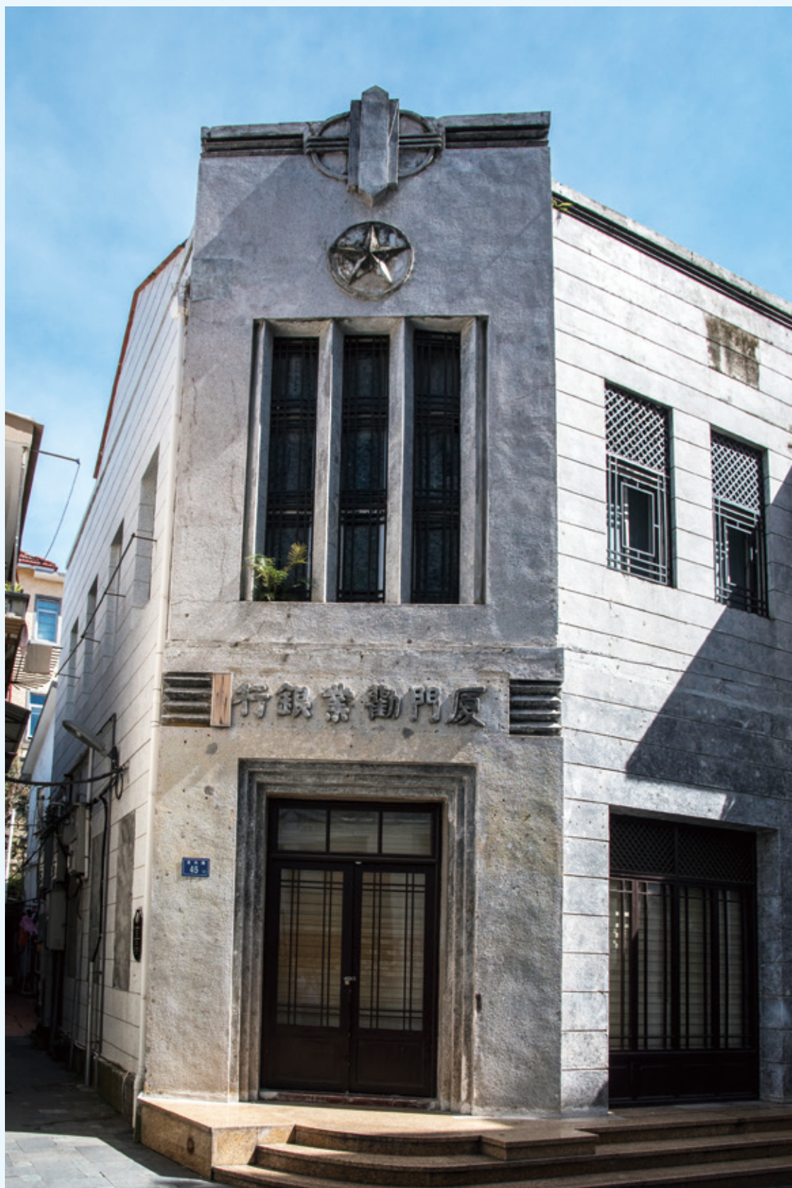
◎ 厦門勸業銀行旧址。(康倫恩 攝) Former Kangyo Bank, Amoy. (Photo by Kang Lun'en)
